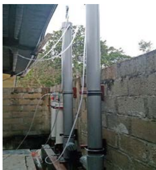
Figure 2. Absorber Column Set-up
