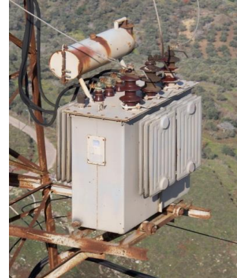
Fig 7: Distribution transformer
